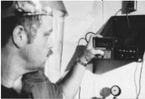
Monitoring pressure and temperature.
